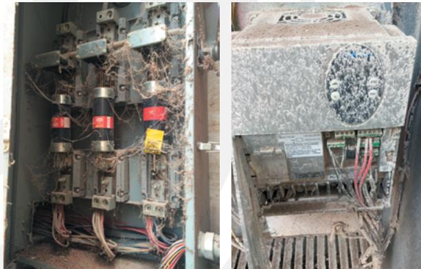
**2** Cleaning is not just about cleaning. A solid EPM program should include de-energized maintenance at least every three years on electrical equipment. The perfect time for routine exercising of your breakers and oiling and lubricating moving parts is while you are already there cleaning during a de-energized state. Cleaning is a great time for getting inside de-energized equipment to check cable connections, wear and tear and torque bus connections.
